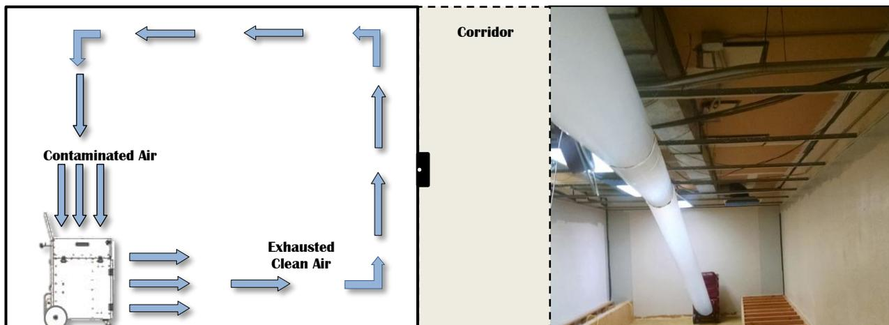
Diagram illustrating the concept of air scrubbing while the photo shows an air scrubber working inside a contained area with a diffuser hose attached to the exhaust. The plastic "lay flat" has been perforated to allow the air to diffuse throughout the room.
