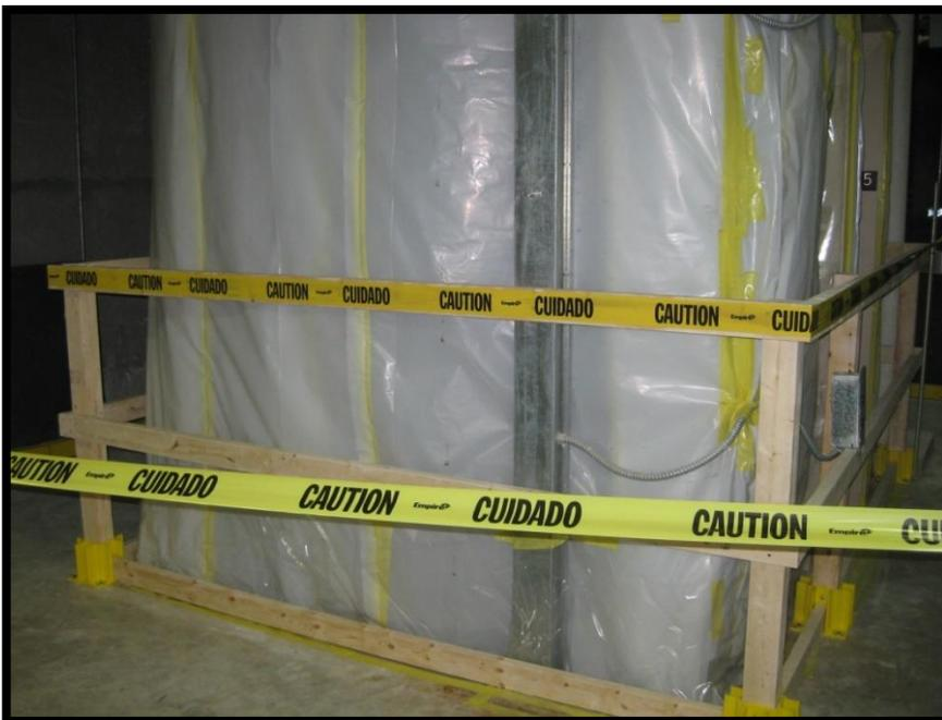
In addition to the mold remediation, extensive safety precautions had been utilized to prevent material, equipment, or individuals from falling into the elevator shaft once the wall materials were removed.
