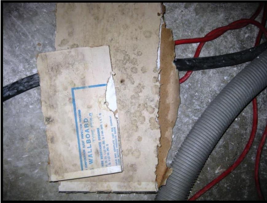
By the end of the project, approximately 115,000 square feet of contaminated gypsum wallboard material and nearly 20,000 square feet of 1" thick elevator shaft liner board had been removed from the tower and replaced with new material.
