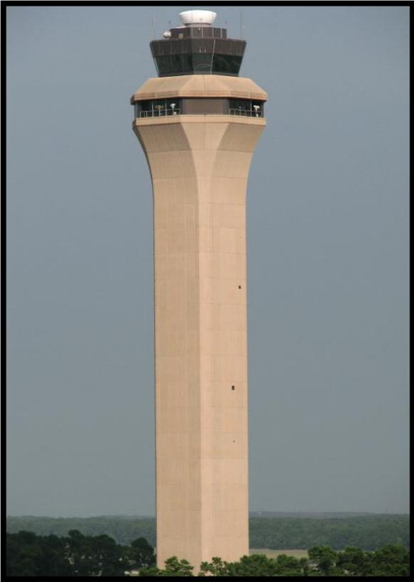
Photo of a typical Air Traffic Control Tower (ATCT) found at larger airports across the US. Most of the windowless square tower is designed to be unoccupied. Radar equipment is on the roof and in the rooms where the tower flairs outward. The air traffic controllers work in the glassed-in section at the top of the tower called the "CAB."
