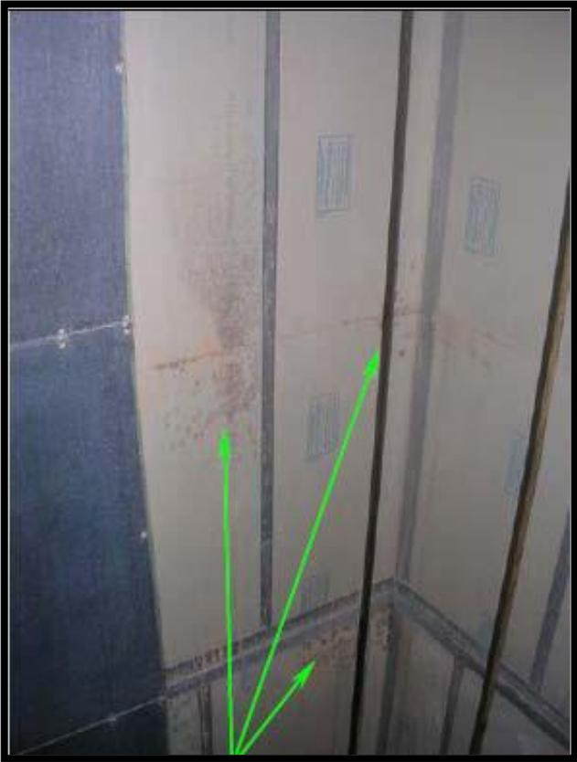
The elevator shaft and finished walls on the exterior of the tower had suffered from water intrusion for years. As a result, mold growth was extensive on all the different layers of the material that made up the walls of the elevator shaft and on the back side of the double-layered gypsum boards which served as fire-rated walls along the exterior of the tower. The arrows indicate significant colonies of fungal growth.
