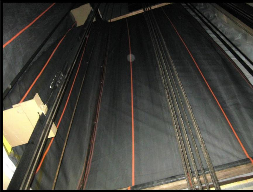
The interior of the elevator shaft was protected on each floor with installation of heavy-duty cargo netting. 20-mil reinforced plastic was sealed to the concrete floors at each level to create an airtight barrier preventing mold contamination from reaching the elevator shaft. The walls of the elevator shaft and liner were then removed from the room side without interfering with the operation of the elevator during peak hours of air traffic.
